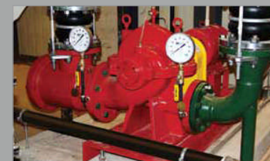
East Hartford High School —EnviroFlo Horizontal Split Case Pumps met critical construction schedule demands with easy, groutless base installation. Now they're providing high efficiency primary/secondary chilled water and condenser water movement for reliable student/teacher comfort.
